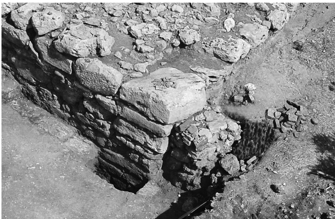
Pl. 29. View of the northwest corner of the Platform from the Northwest, showing wall CT-058.
