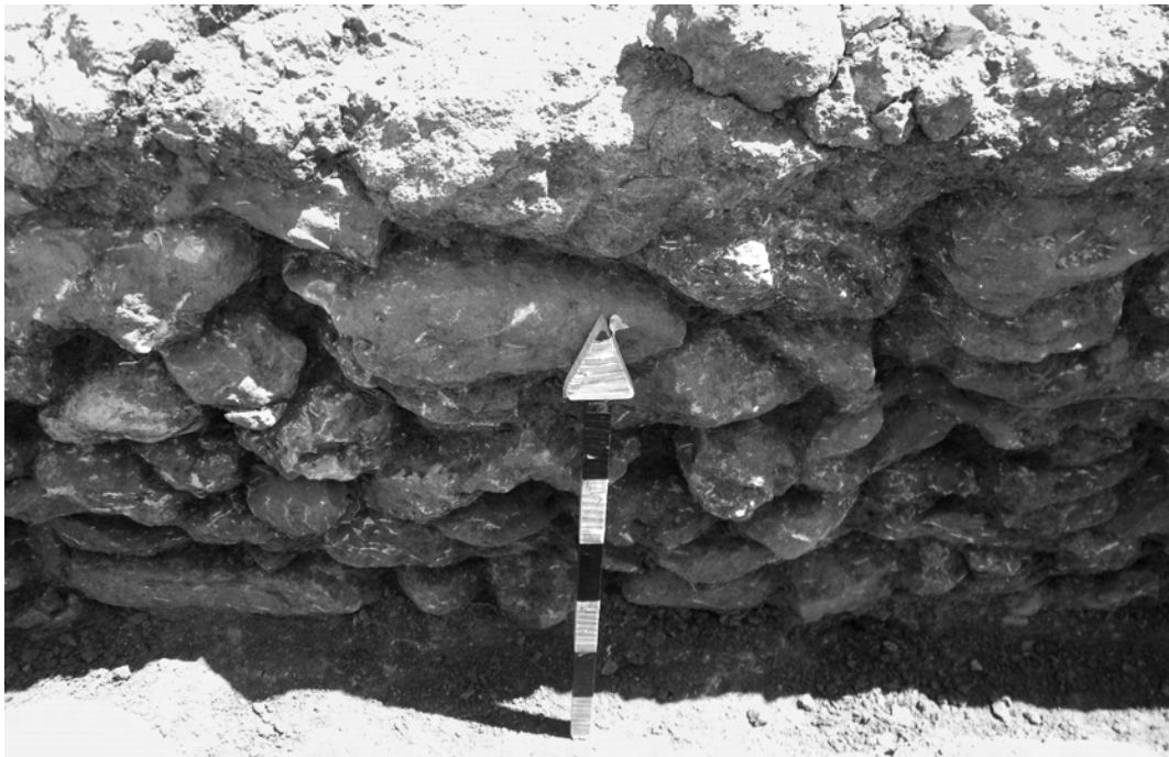
Pl. 130. The southwest wall of drain ζ.
