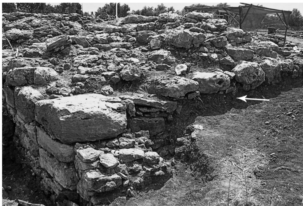
Pl. 9. View of the west face of the Platform from the West. The arrow indicates the layer of skarmigia under the Cyclopean blocks of the west side.
