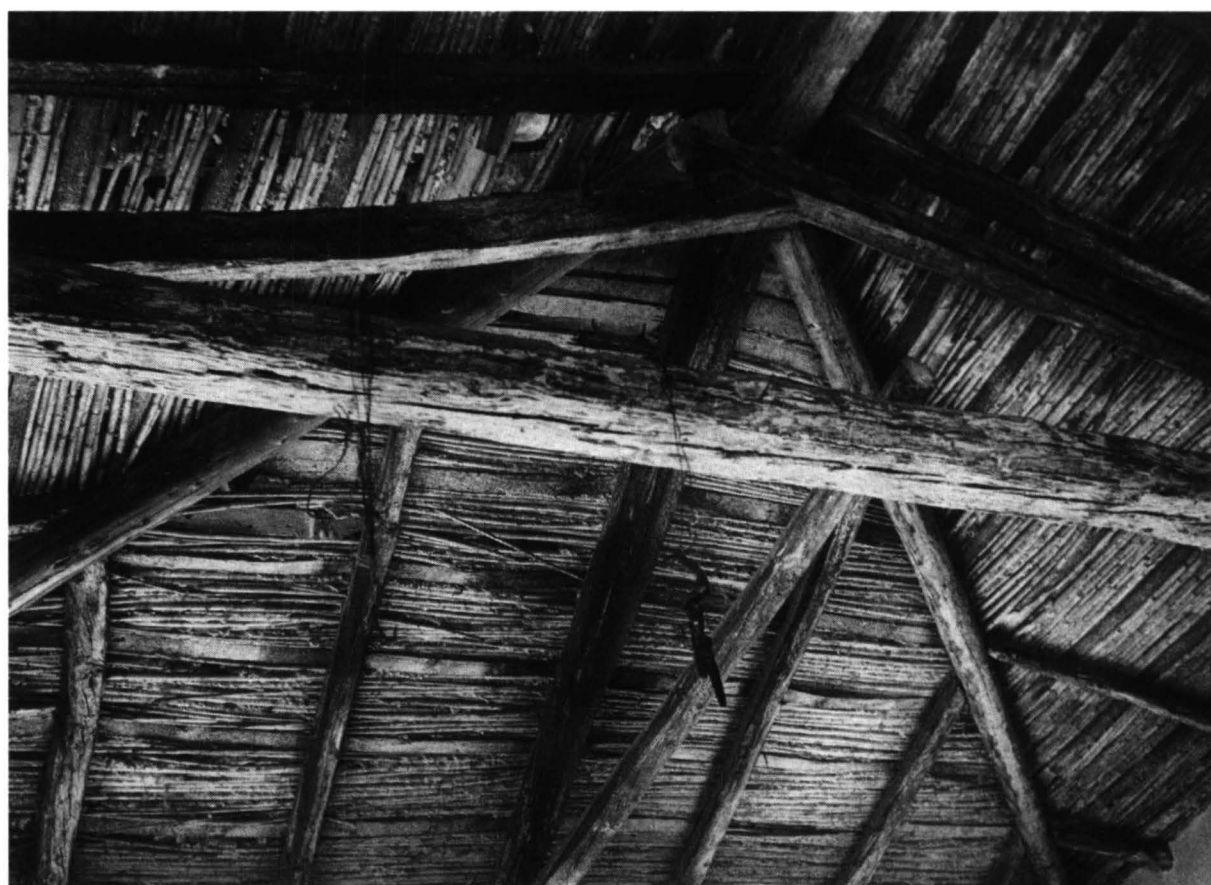
185. Sheathing of reeds supporting clay bedding for roof tiles (house in modern village of Mycenae).
