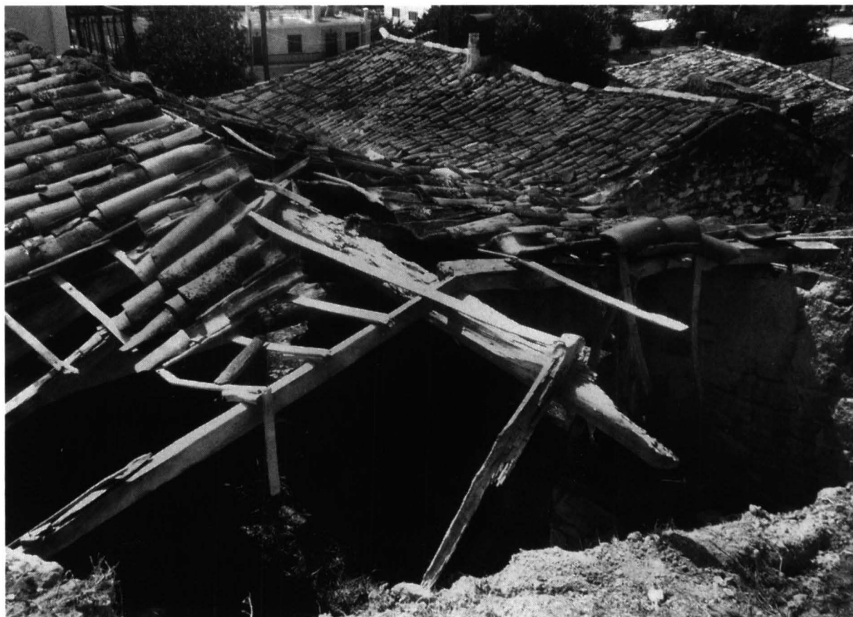
184. Roof tiles arranged straight on lattice of laths, without clay packing (house in modern village of Mycenae).
