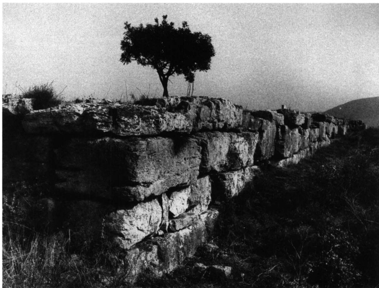
34. Melathron, east retaining wall with offsets.
